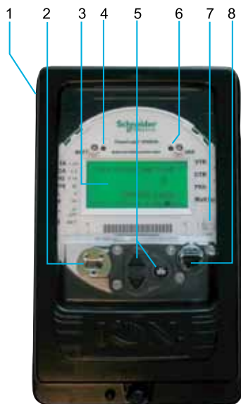
PowerLogic ION8650 switchboard meter.
